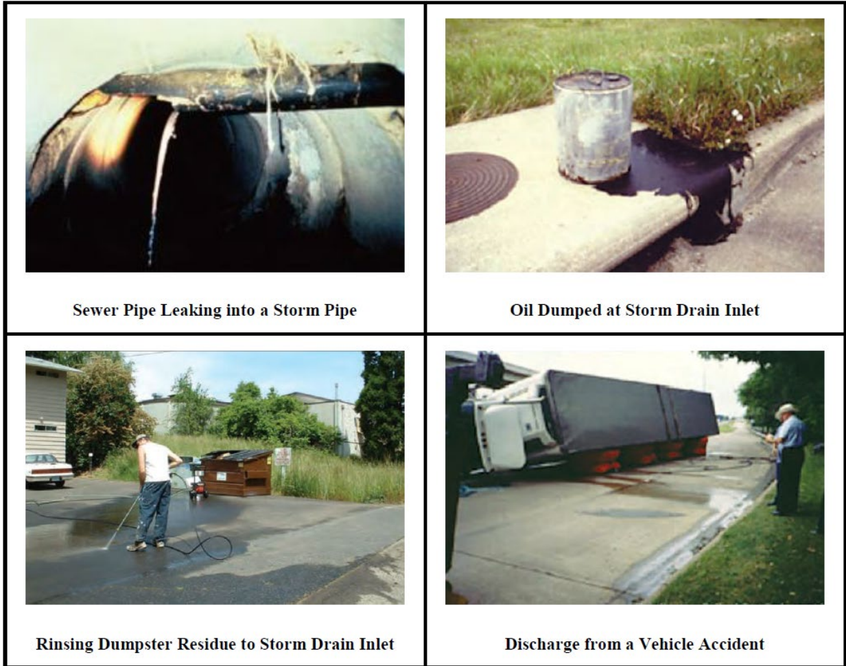
Figure 1. Examples of Illicit Discharges
